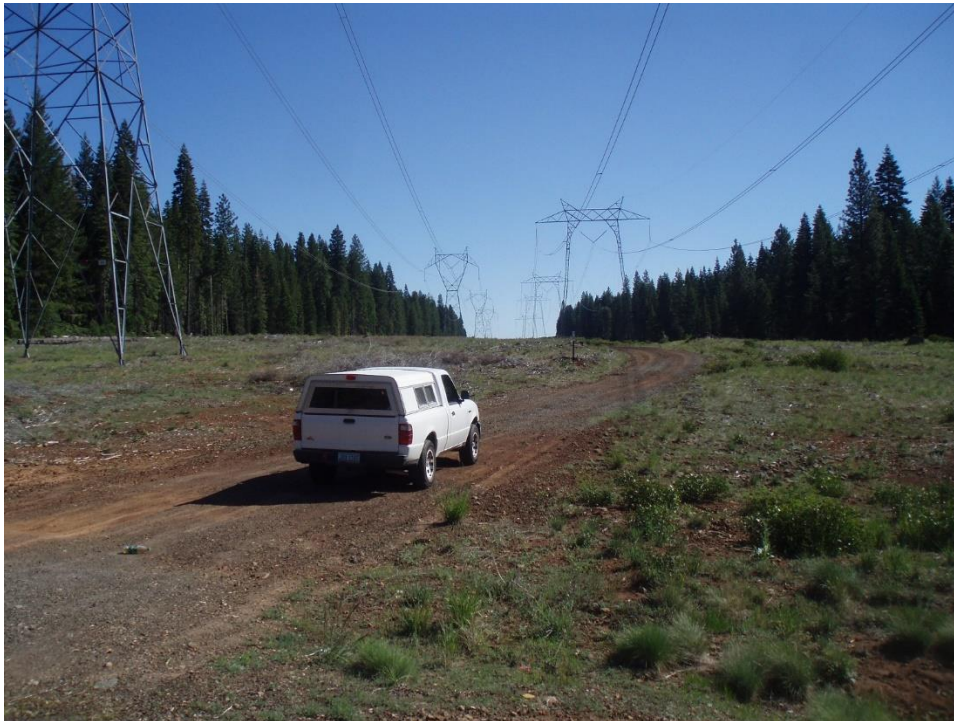
Vegetation control and service road associated with twin extra-high-voltage lines.
